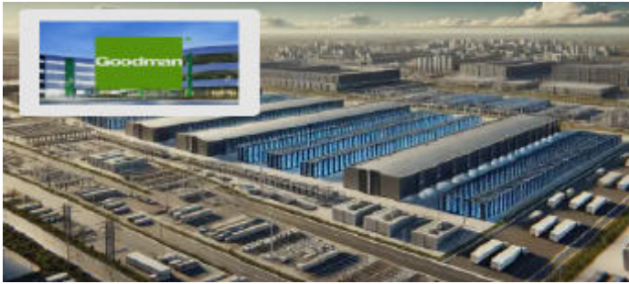
Goodman Craigieburn Melbourne Data Centre in Craigieburn, Victoria. Pic: Datacenters.com
